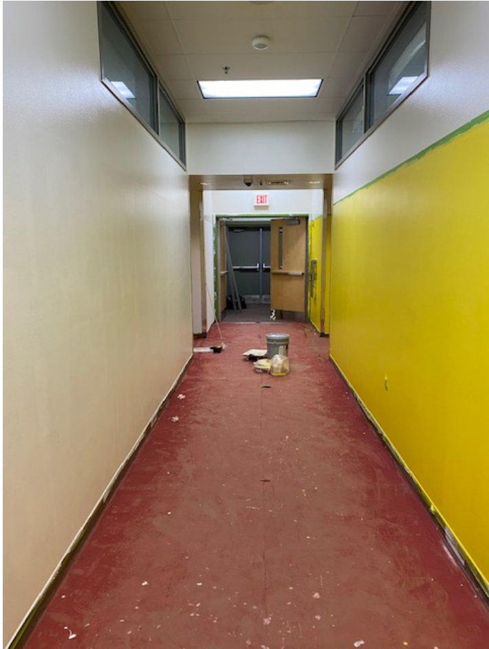
3 rd Coat of Cream & 1 st Coat of Yellow
