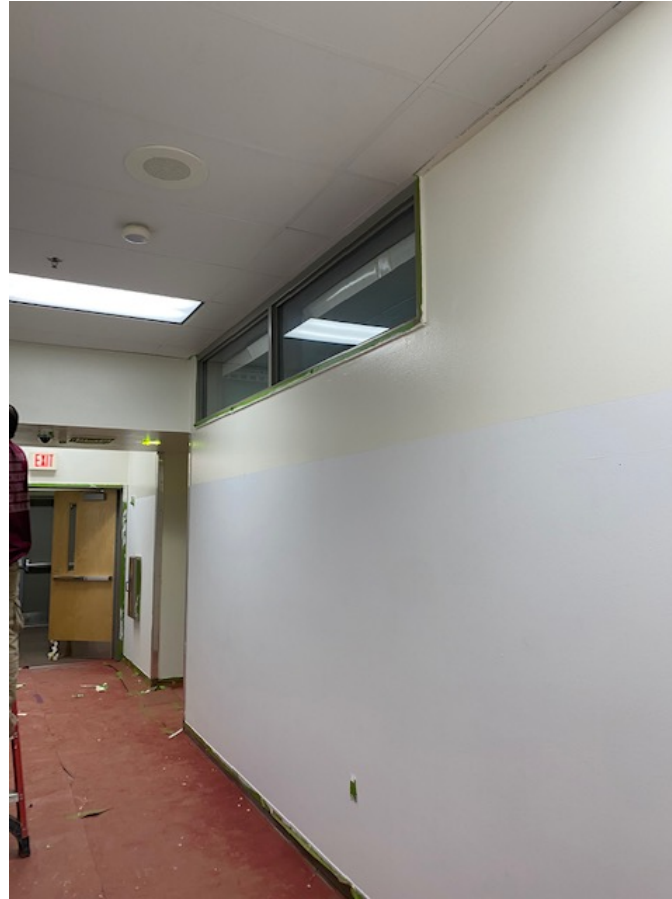
1 st Coat of Cream Paint
