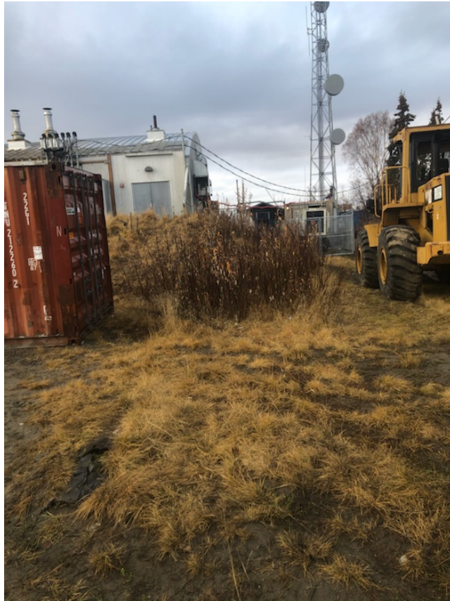
New prime power JD replacement generator in connex. Delivered by Crowley.
