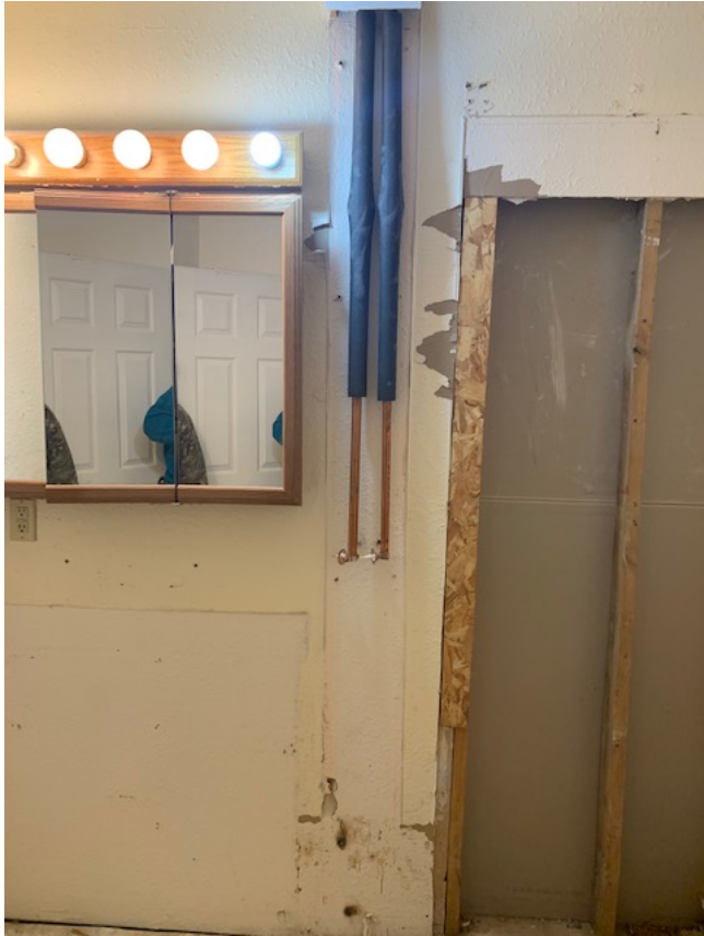
Demolition of bathroom
