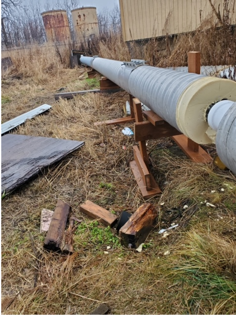
Repaired Dip in the line & Rebuilt the Pipe Stand
