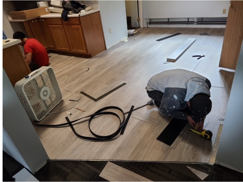
Training on Floor Coverings Installation
