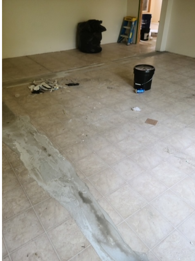
Prepping the floor, removing cracked loose vinyl, ardex to level the floor for installation of new LVT
