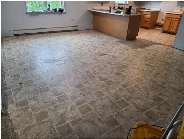
Previous flooring with holes, being filled with ardex for leveling
