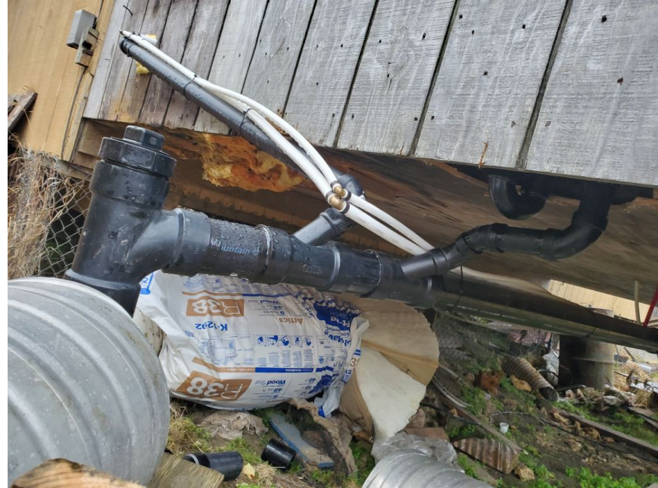
New Water & Sewer Line Ready for New Utilidor & Heat Trace.
