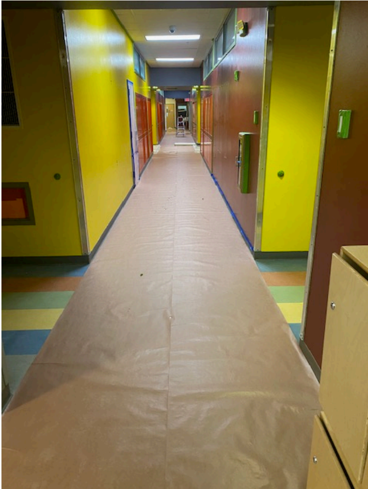
Prior to Repairs
