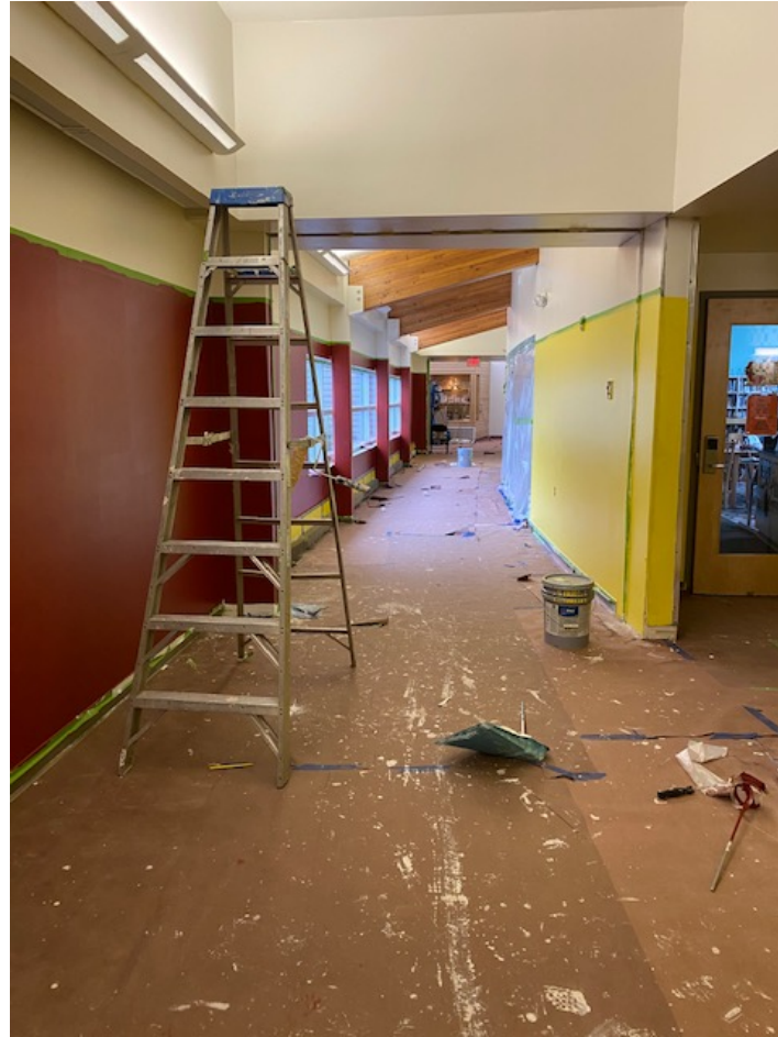
Final Coats of Paint
